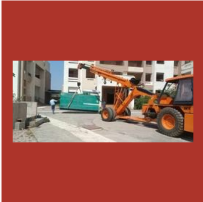
Diesel Generator in Iran
