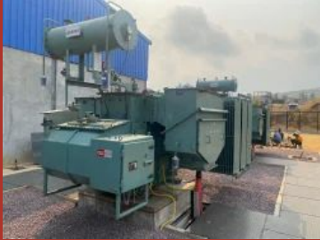
200 KVA 3 Phase Distribution Transformer
