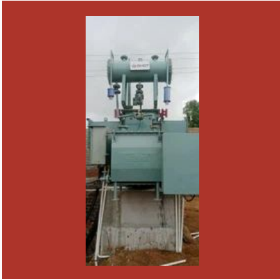
Top 10 Diesel Transformer Dealers & Suppliers In Dubai
