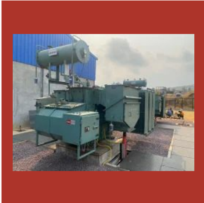
500Kva 3-Phase Distribution Transformer
